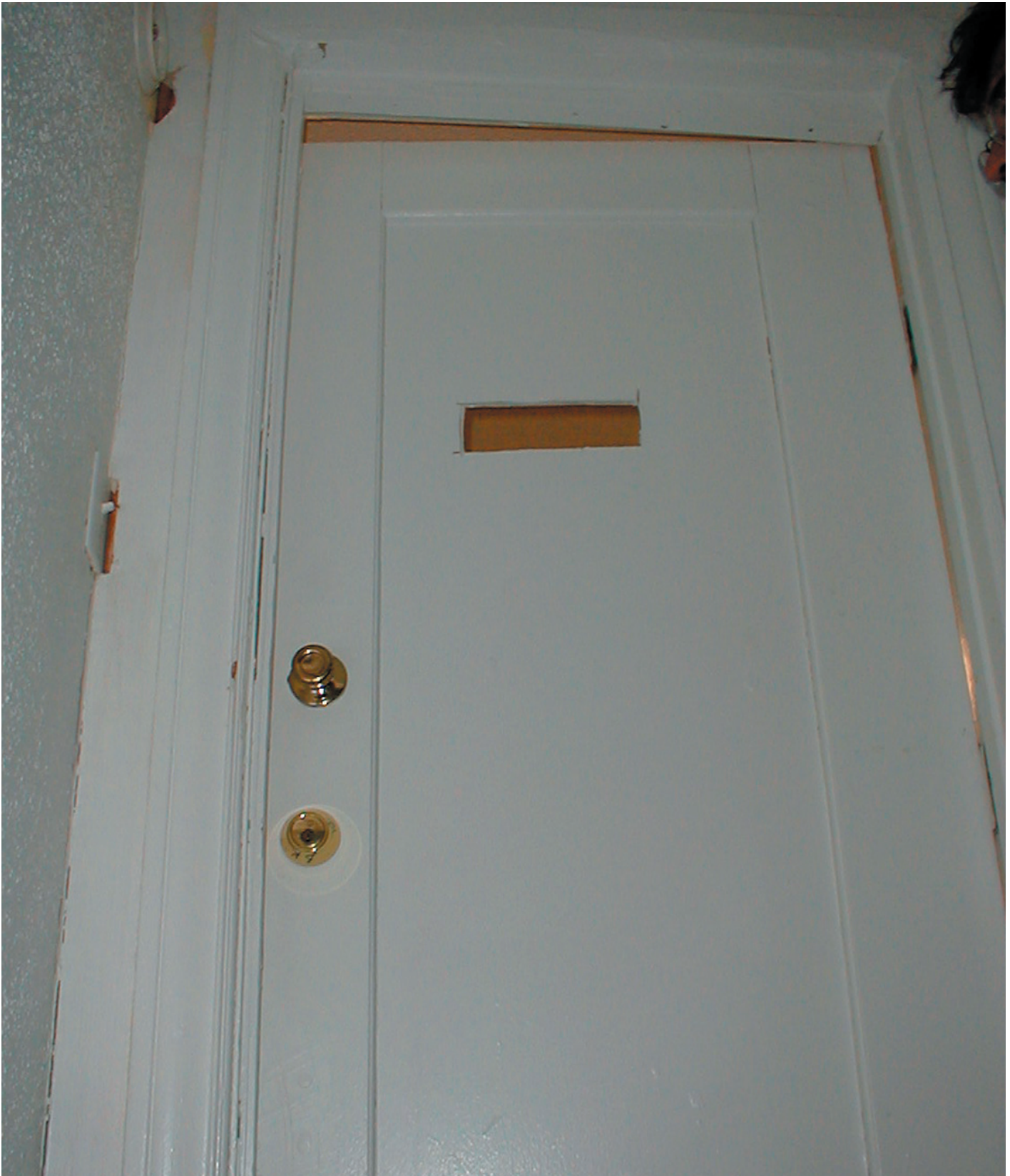
Peephole on door of attic room at a residential treatment center.
